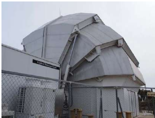
Figure 77 - The segmented roof of the Faulkes South Telescope (Context 2014).
