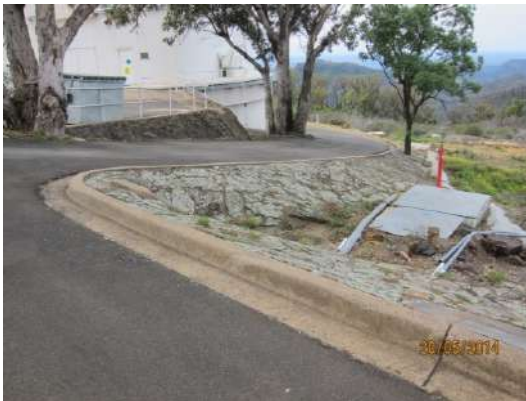
Figure 87 - Crazy paving between the 24 Inch Telescope and the ATT (Context 2014).
