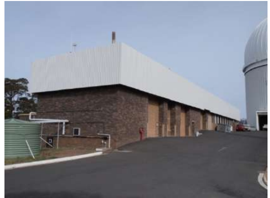
Figure 60 - The Workshop building with the AAT at the right of picture (Context 2014).
