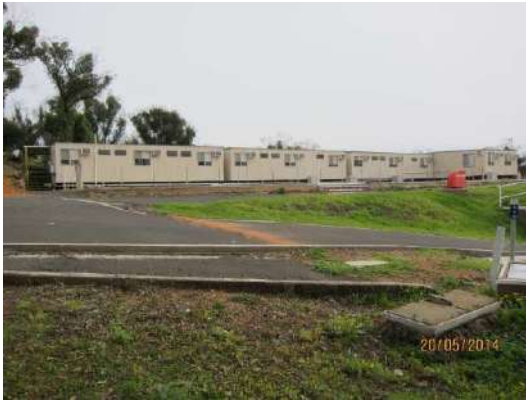
Figure 67 - The demountable temporary accommodation currently occupying the lodge site (Context 2014).
