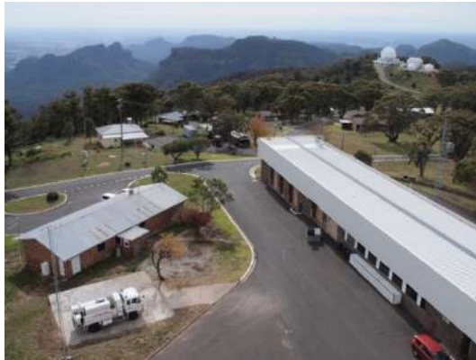
Figure 59 - Administration Precinct with the Workshop on the right and the Administration Building on the left. The site of the Fire Station is in the left foreground and the Residential Area and Eastern Telescope Area in the background (Context 2014).
