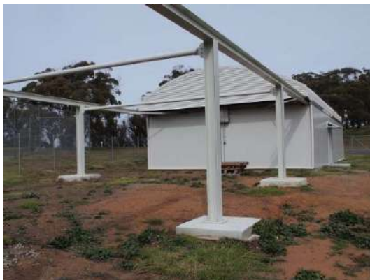
Figure 79 - The utilitarian design of the iTelescope building, showing the frame onto which the roof slides when opening (Context 2014).
