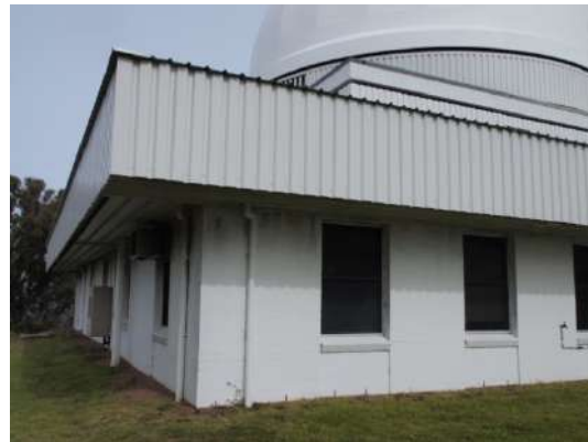
Figure 84 - The deep eaves of the UK Schmidt Telescope building – compare with Figure 83 (Context 2014).
