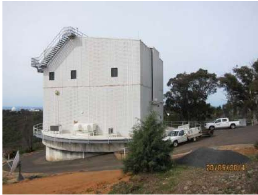
Figure 75 - The 2.3m ATT structure, the whole of which can be revolved on its circular concrete base (Context 2014).
