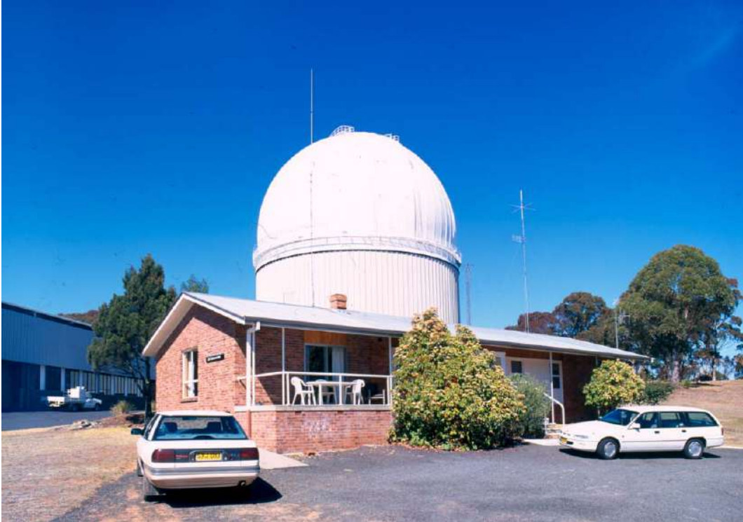
Figure 35 - Looking south at the Administration Building at its current extent. To the left is the Anglo-Australian Workshop, with the Anglo-Australian Telescope in the background (exact date of photo not known) (ANU RSAA Archive, accessed August 2014).
