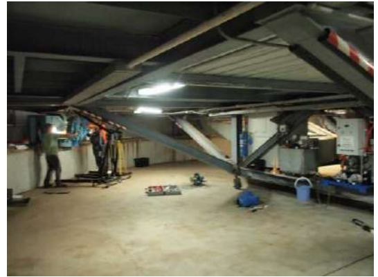
Figure 76 - Showing the truss floor and mechanised bogeys (under repair in the image) which enable the 2.3m ATT structure to be rotated (Context 2014).
