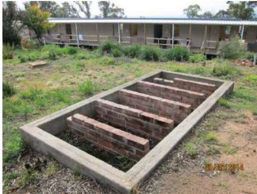
Figure 91 - Concrete and brick structure which probably supported a tank or generator relating to the Lodge destroyed by the 2013 bushfires (Context 2014)
