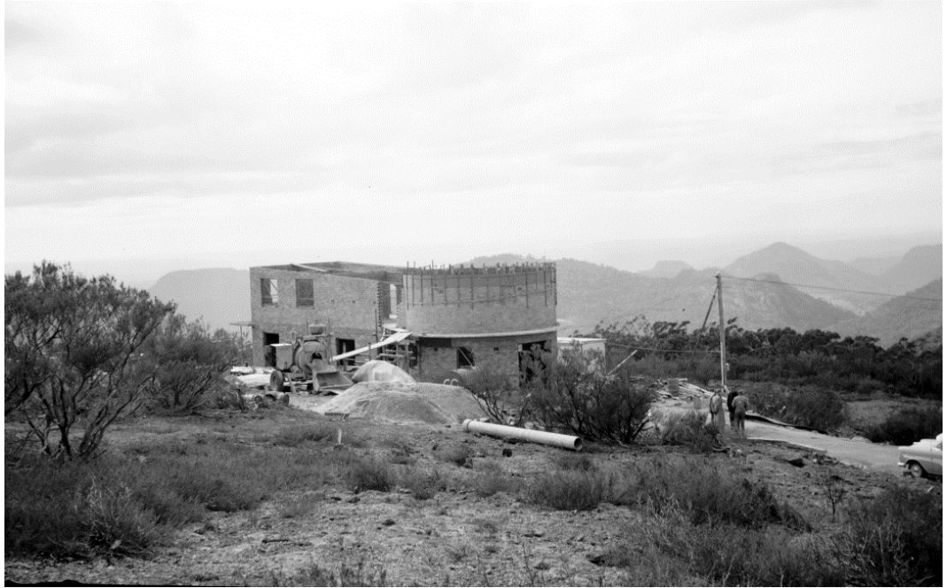
Figure 14 - The construction of the building to house the 40 inch telescope – the first telescope installed on site, which was officially opened in 1964 (ANU RSAA Archive, accessed August 2014).
