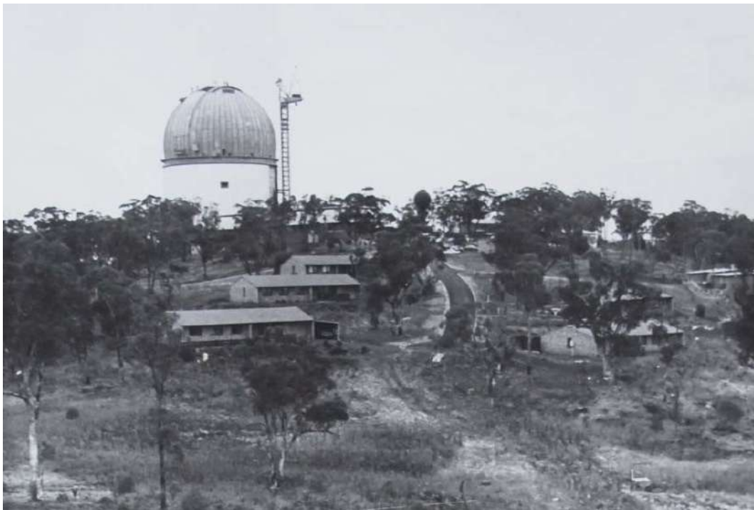
Figure 21 - A photo dating to c1973, looking south west to the Anglo-Australian 150 inch Telescope during construction, and showing the residences in the foreground (Judy Over photo collection).
