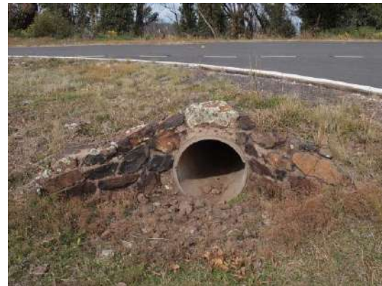
Figure 88 - Culvert under Observatory Road to the south of the Faulkes Telescope (Context 2014).
