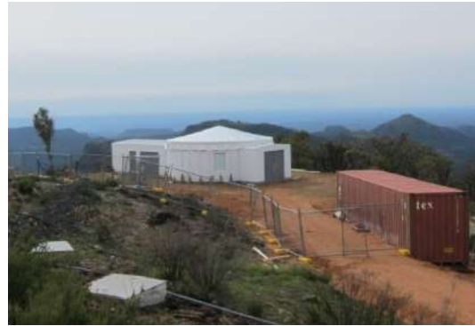
Figure 82 - The KMTNet Telescope under construction, showing the central telescope enclosure and adjoining annex (Context 2014).
