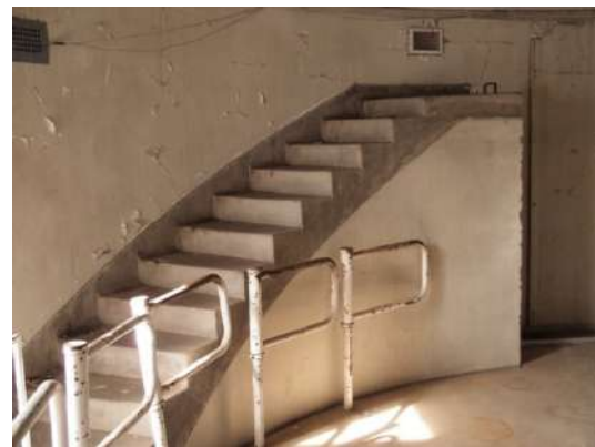
Figure 74 - Staircase and barriers within the viewing chamber for the 40 inch Telescope, designed to enable access to the telescope and as a safety precaution when the floor was hydraulically raised (Context 2014).
