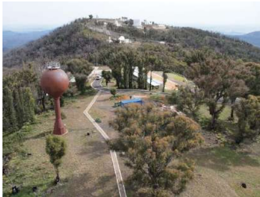
Figure 65 - View north west from the external walkway around the dome of the AAT (Context 2014).
