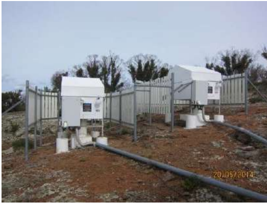
Figure 81 - The basic telescope casings of the remotely operated HAT South Telescope structures (Context 2014).
