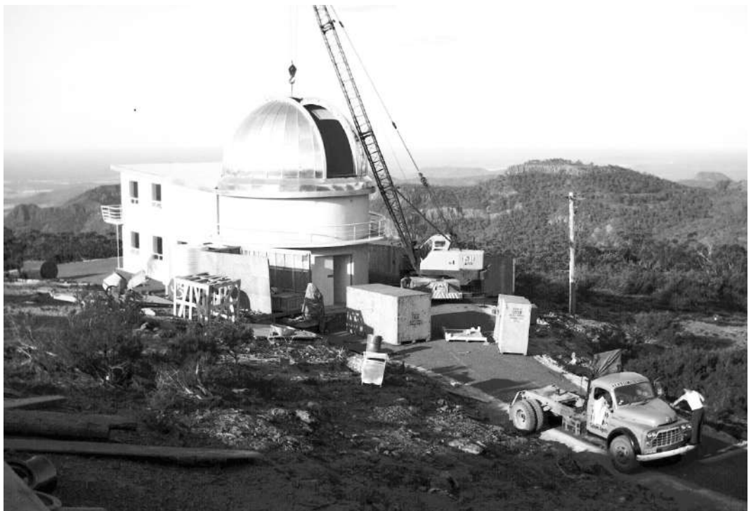
Figure 15 - The dome being installed on the 40 inch telescope building, in 1963-4 (ANU RSAA Archive, accessed August 2014).
