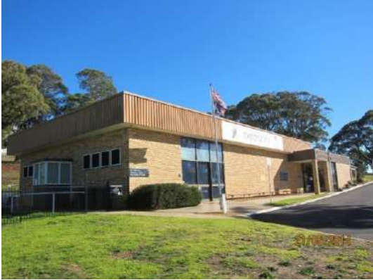
Figure 57 - The Siding Spring Exploratory/Visitor Centre from the south east (Context 2014).
