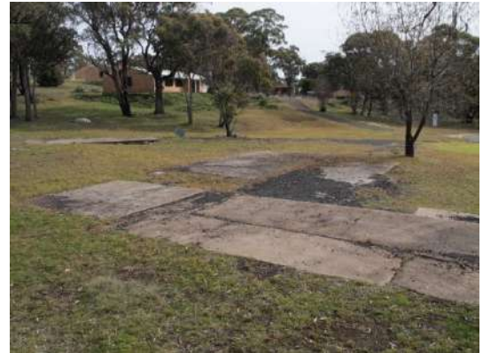
Figure 92 - Concrete pads to the south of the Tennis Court representing the site of a group of now demolished houses
