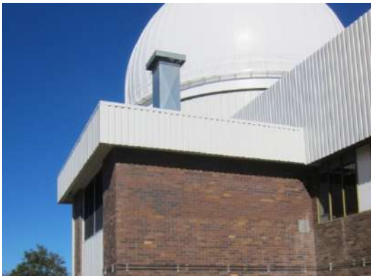
Figure 83 - The deep eaves of the Workshop buildings – compare with Figure 84. AAT in the background (Context 2014).
