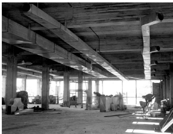
Figure 3.7: The air-conditioning system was designed for the original configuration of the building. The system has been re-balanced a number of times to account for the change of use in certain areas and the diminishing book stock, which acted as a 'heat-sink' for the building (ANUA15 111 – UN343/14 1965)
