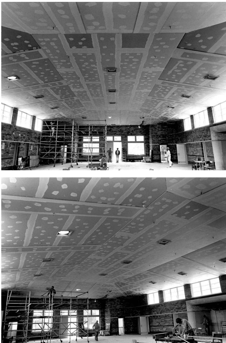
Figure 3.5: False walls and ceilings were added to the building when it was converted into an art gallery in the mid-1980s (Sept 1984, ANU Archives).
