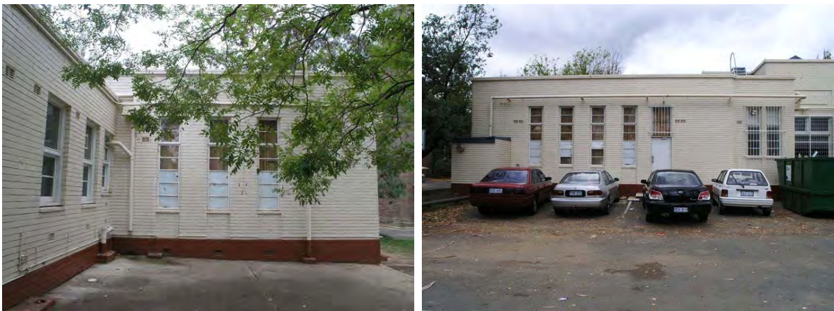
Figure 4.7: Windows and downpipes of the northeast corner
