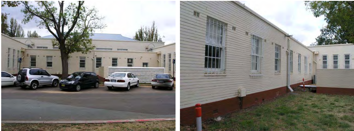
Figure 4.8: The window grilles and air cond. unit enclosure of the west side of the building
