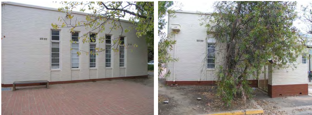
Figure 4.6: Windows and air-con. unit enclosure on the southeast corner
