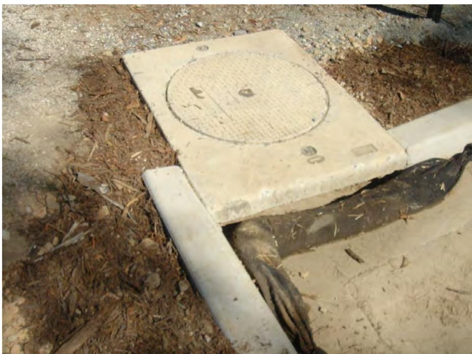
**Figure 5.3. Partial failure of stormwater drain protection at construction site.**
