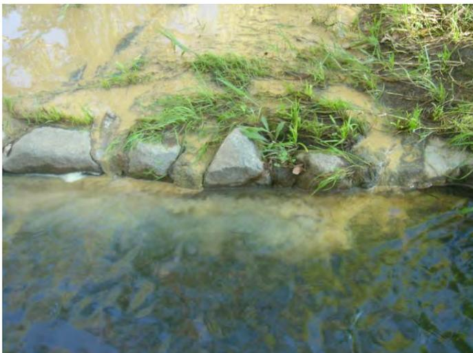
**Figure 5.2. Sediment load entering Sullivan's Creek through stormwater drain from construction site**
