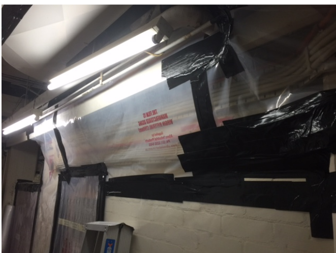
Encapsulation of internal fittings
