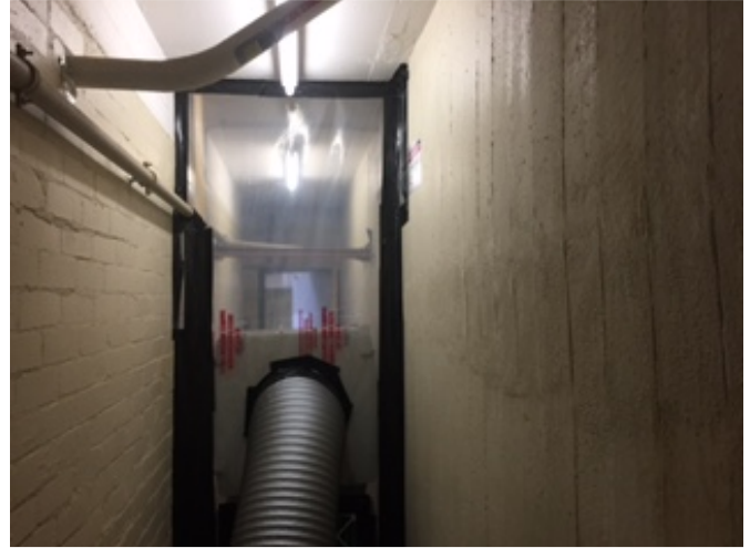
Negative pressure units end of enclosure
