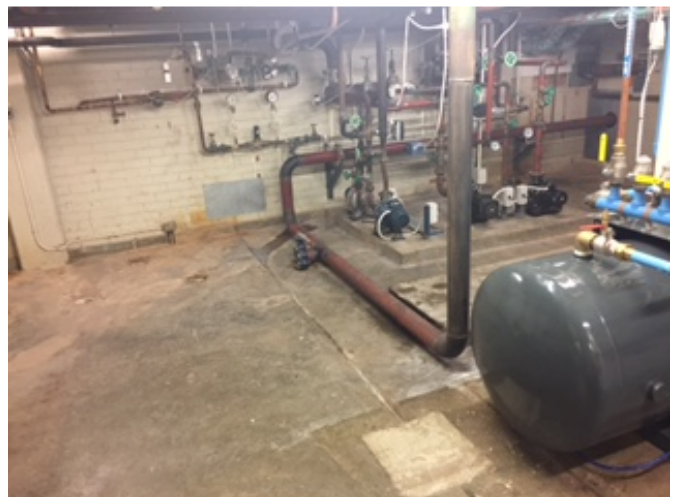
Removal Area - Stage 2
