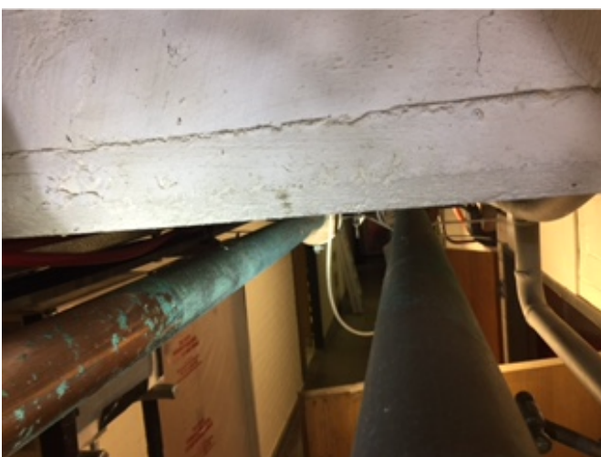
Removal Area - Stage 2
