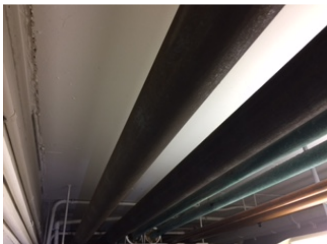
Removal Area - Stage 2
