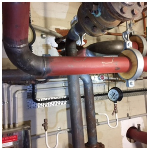
Removal Area - Stage 2
