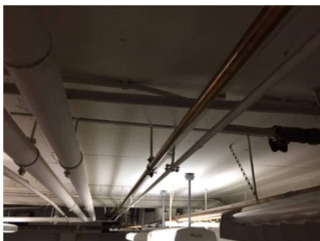
Removal Area - Stage 2
