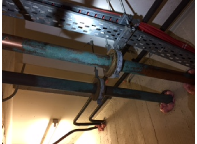
Removal Area - Stage 2
