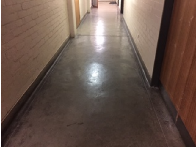
Removal Area - Stage 2
