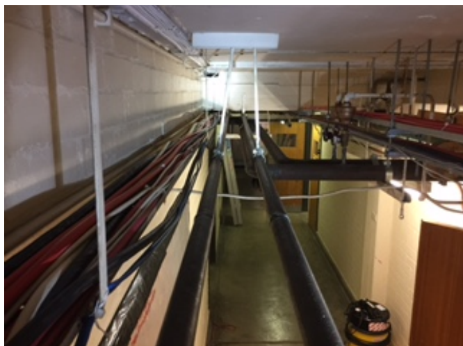
Removal Area - Stage 2
