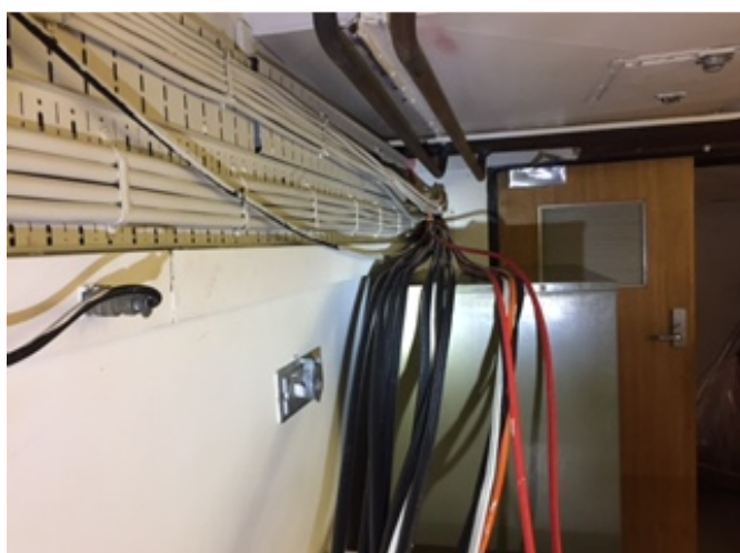
Removal Area - Stage 2
