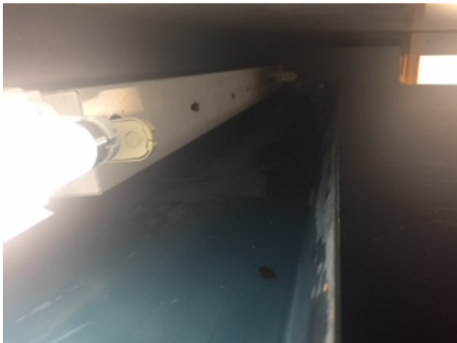
Remediation area - Lift
