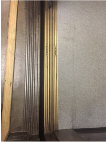
Remediation area - Lift
