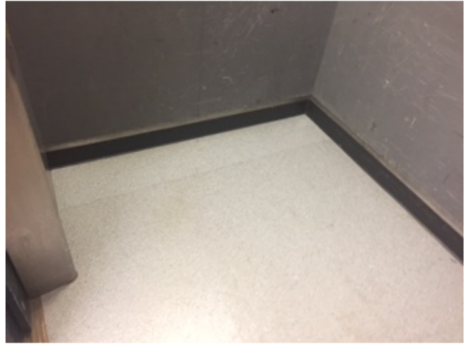
Remediation area - Lift
